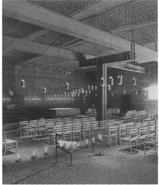
Fig. 12. Interior of St Petri, Klippan, with its cross support
